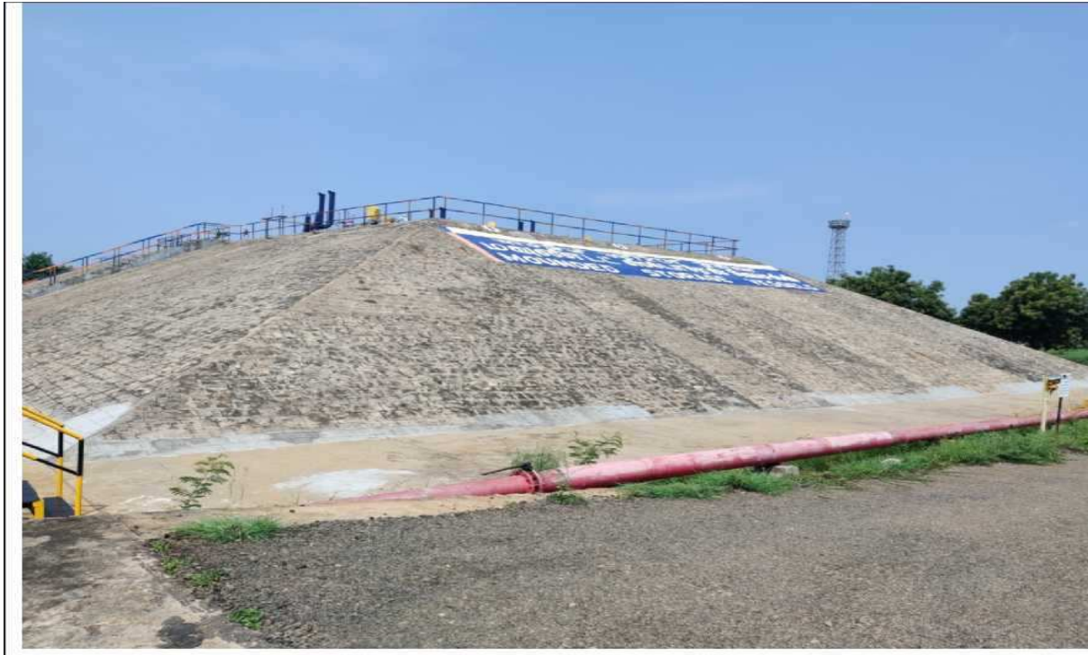
Mounded Storage vessels
